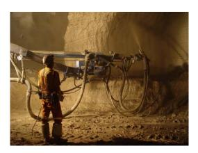
Dosage rate for TYTRO SA 530 depends on cement type, cement content, water-cement ratio, temperature of the concrete, ambient temperature and temperature of the substrate on which the concrete is to be applied. It is always recommended to conduct pre-construction trials to adapt the dosage rates to the properties of the material used and job conditions.
